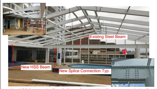
New HSS Beam and a Typ. Splice to Connect New Structure to existing Steel Beams.
